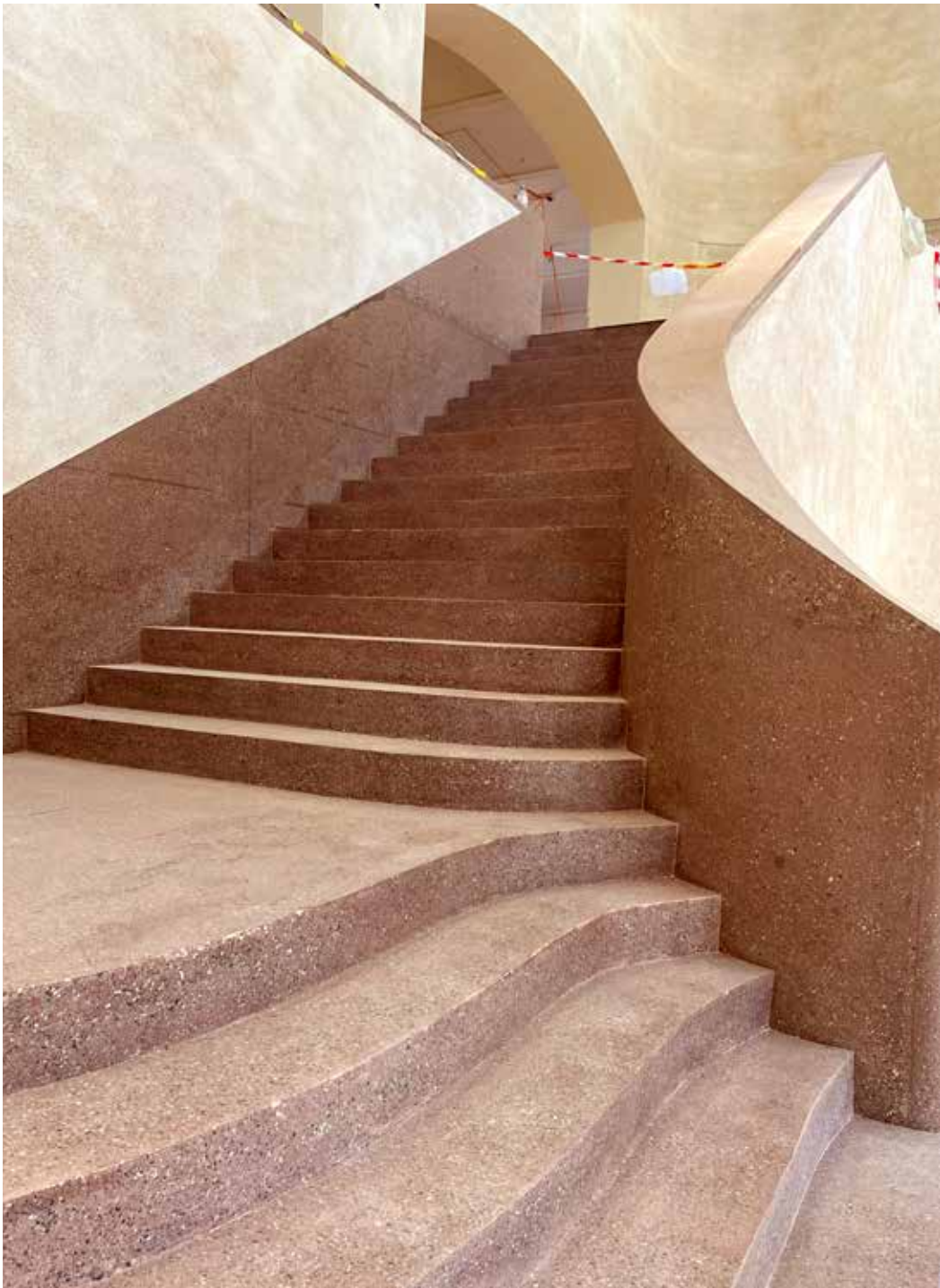
Baustelle - August 2021 Plaza
